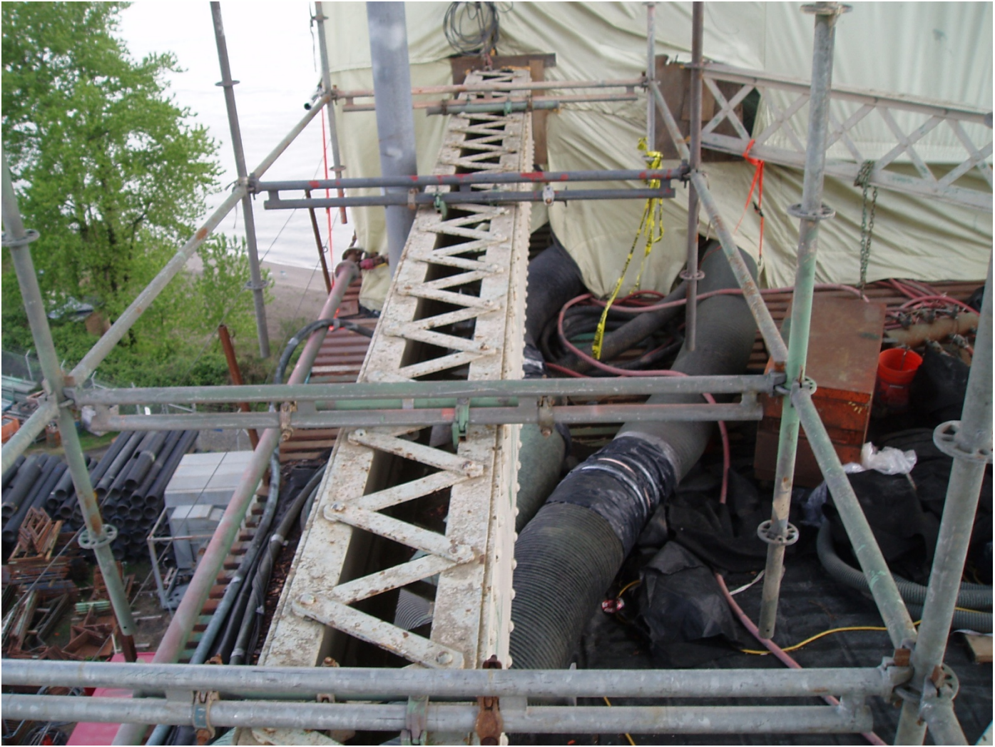
Etobicoke Scaffold Containment Enclosure Attachment To Bottom Truss Chord
