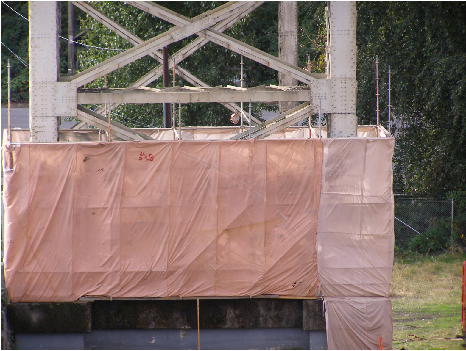
Etobicoke Scaffolding Enclosure Around Pier 6
