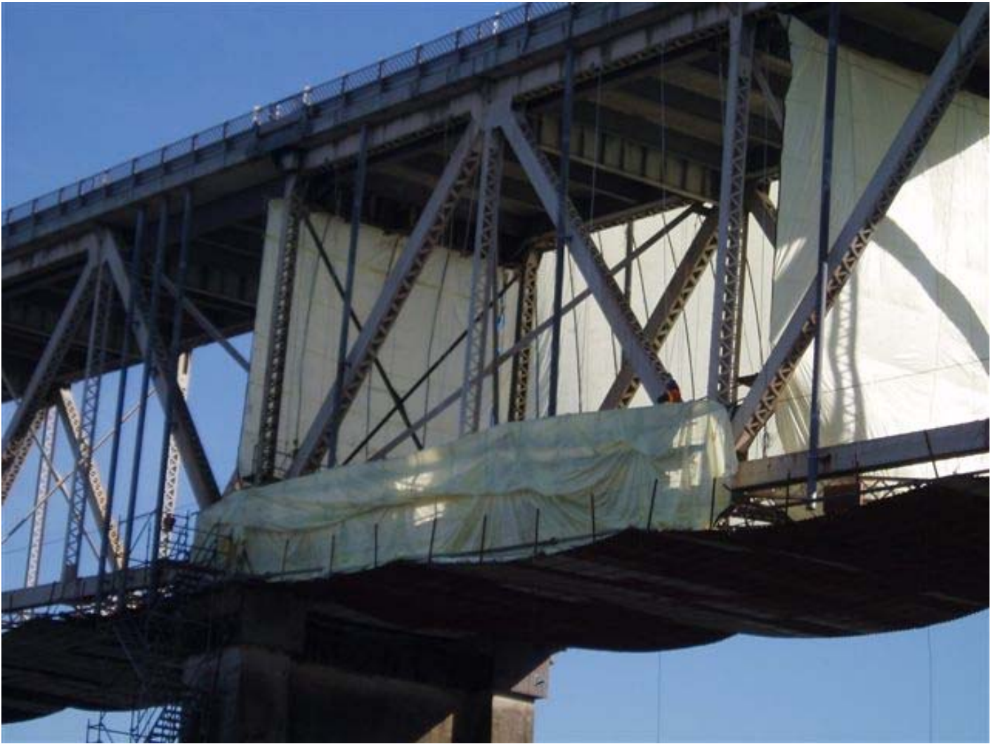
Cable Supported Metal Deck Platform System & Containment
