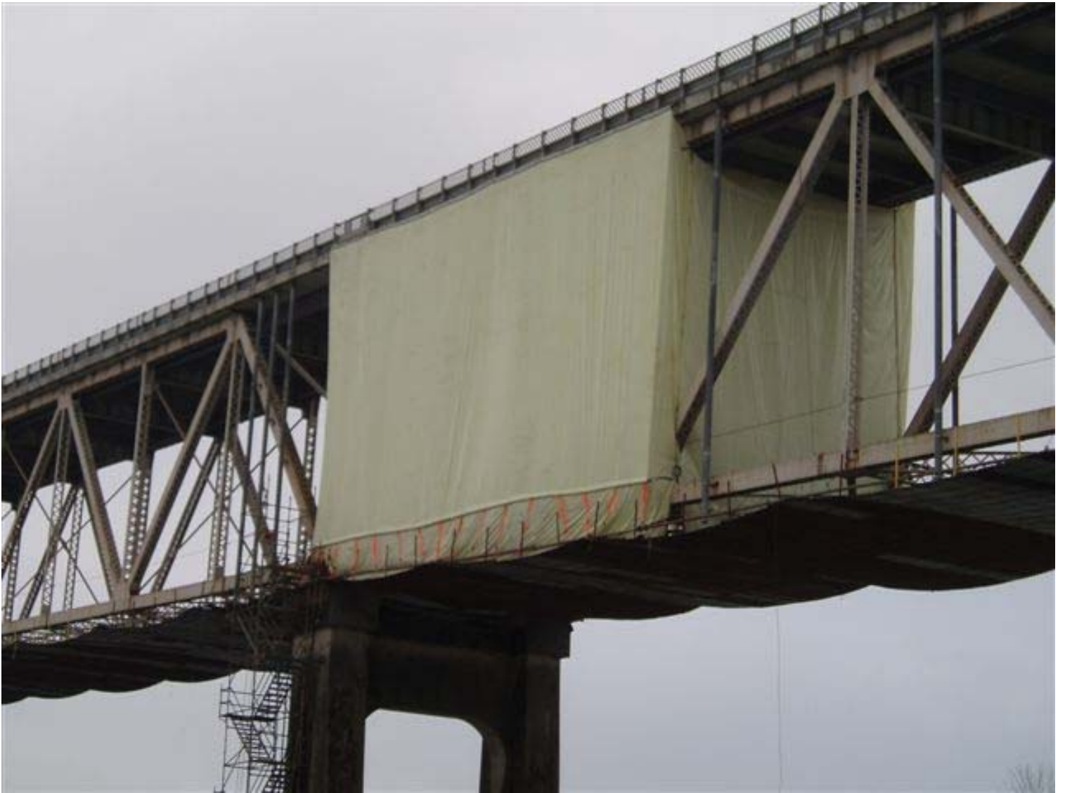
Cable/Metal Deck Platform & Containment W/Scaffold Tower Stairway Access
